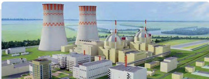
Rooppur Nuclear Power Plant
